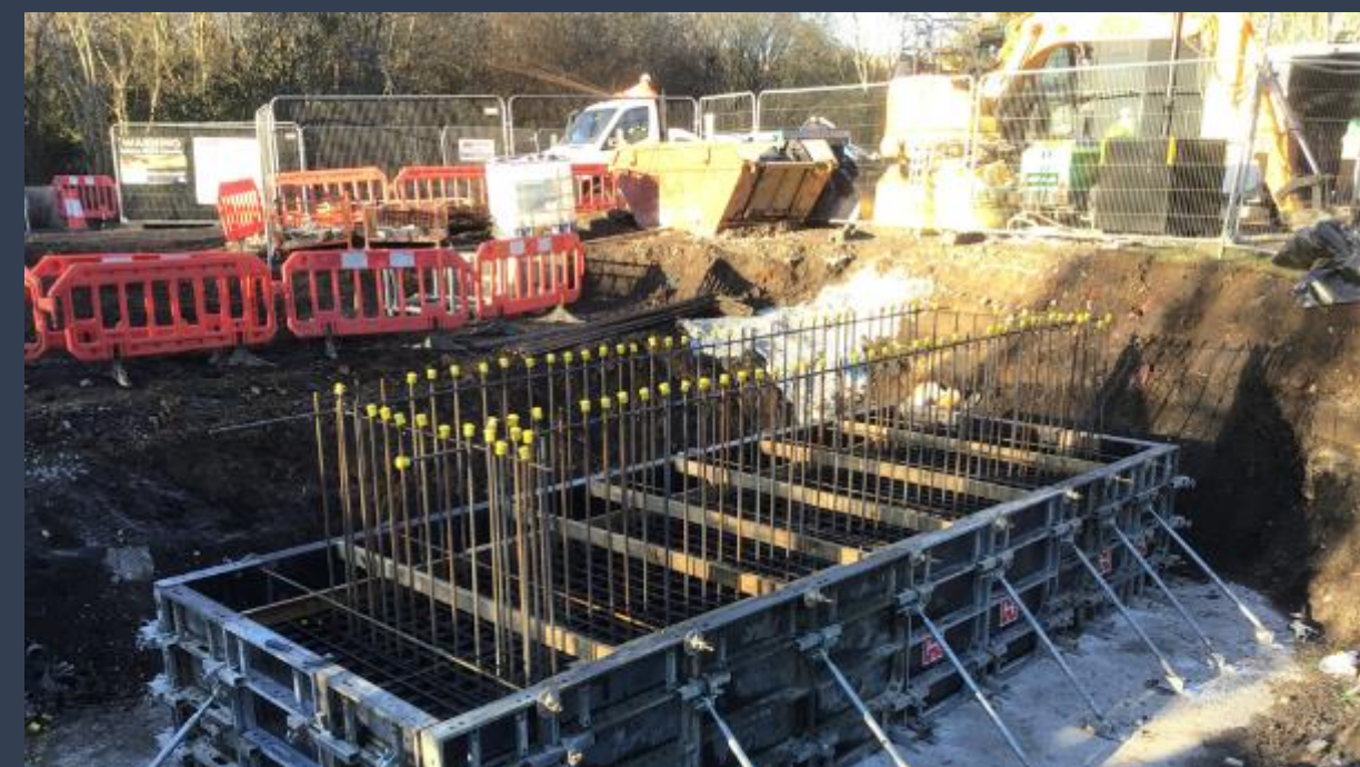
Roch Valley Greenway Crossing under construction – providing a crossing over the river for pedestrians, cyclists and horses.
