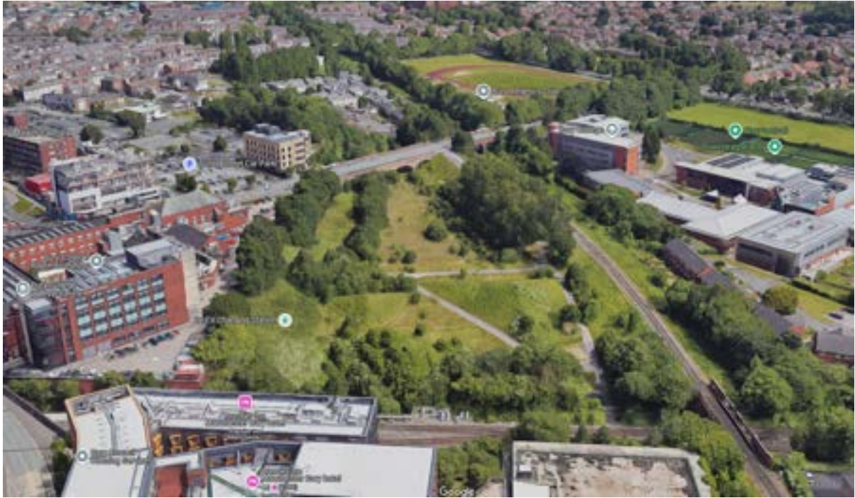
Photo 5 – Aerial from the west
