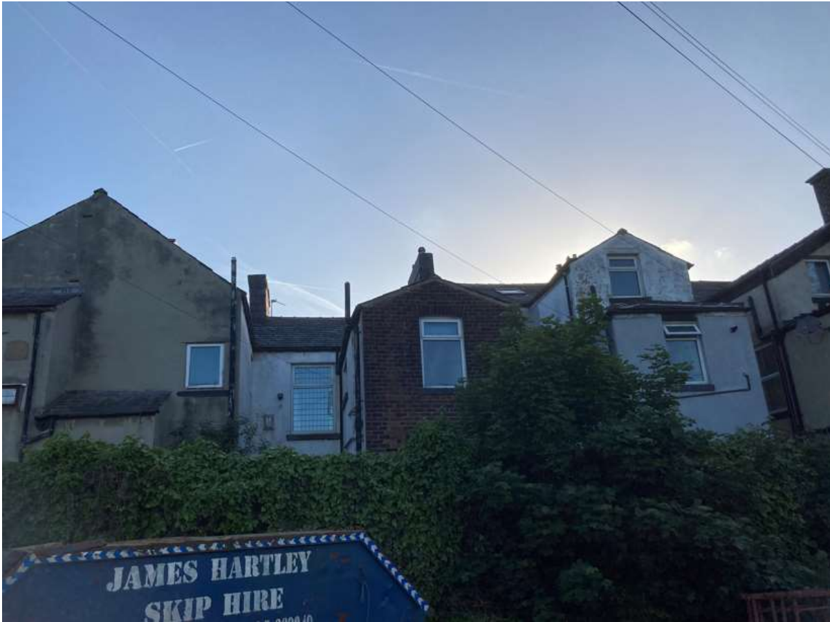
Photo 7: View of rear elevation of application site from adjoining site
