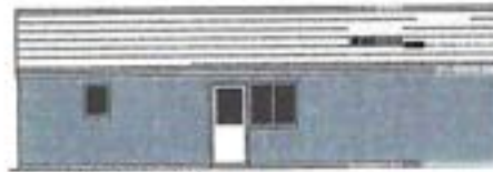
rear - facing south
