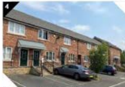
New dwellings at Bridgewater View
