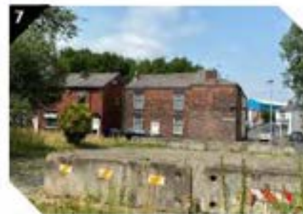
View across to Howard Street from Cuncilffe Street
