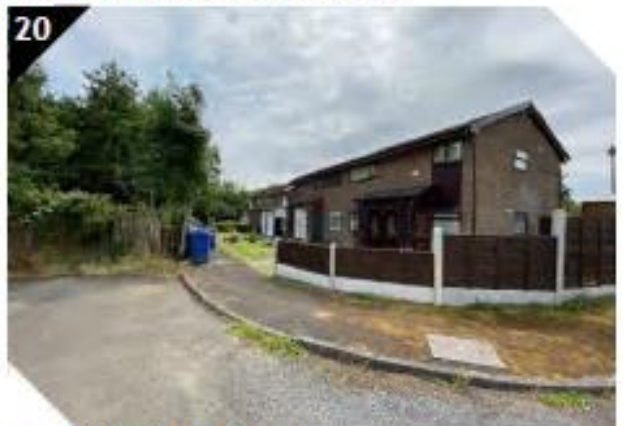
20 Terraced housing at Tower Street
